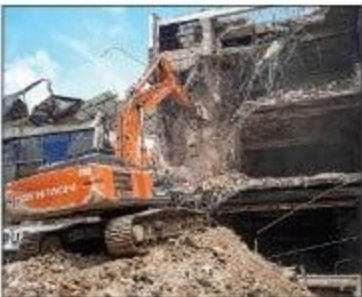
Lucknow Development Authority demolishes the fire-hit building in Aliganj on Saturday. (PTI)
