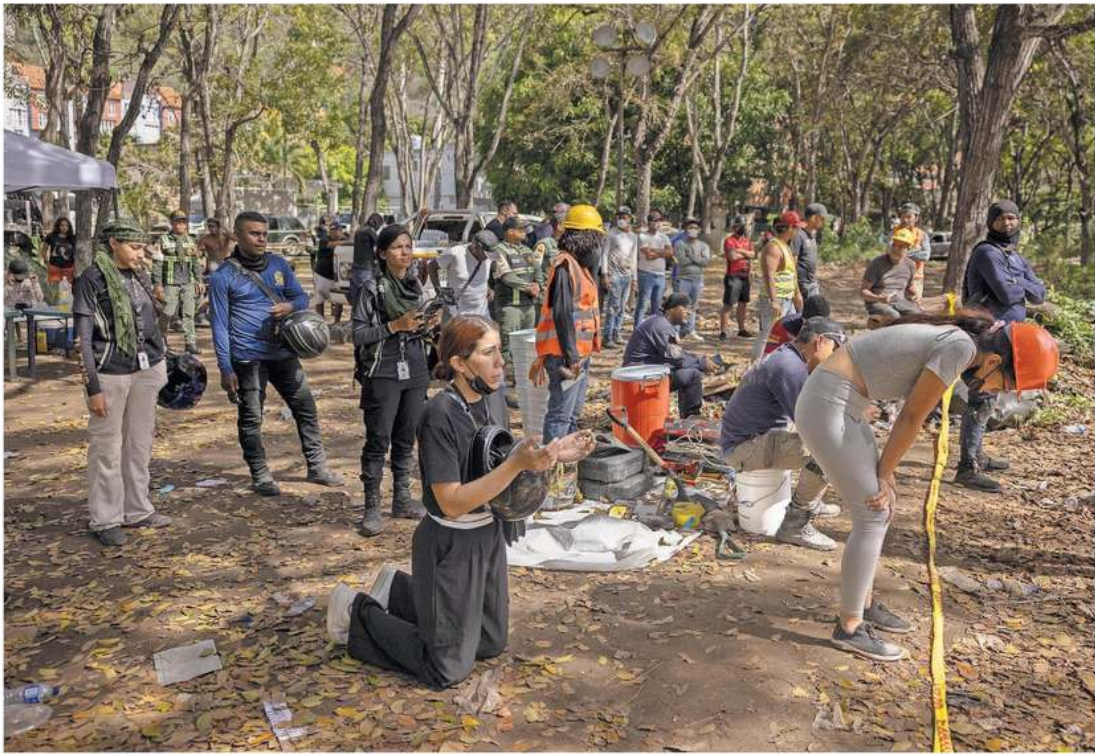
Praying near a collapsed building where rescuers were working last month in La Guaira, the Venezuelan coastal state hit hardest by back-to-back earthquakes in June.
